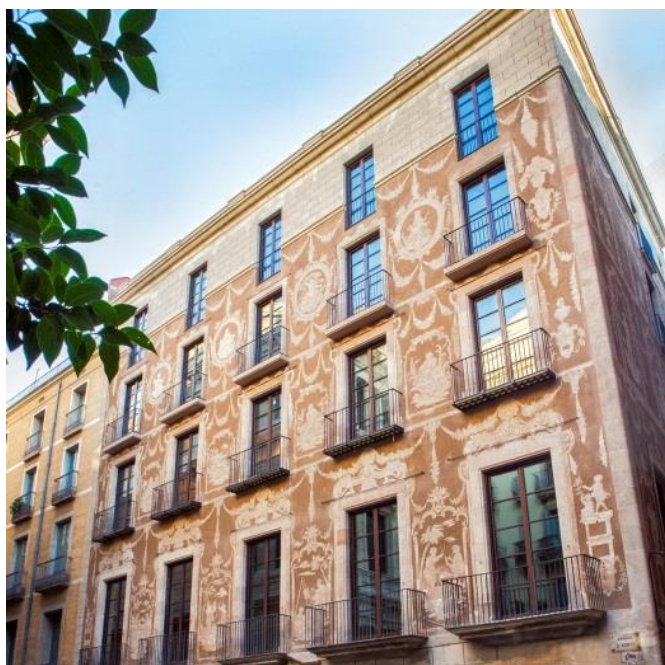
Façade of the Hotel Arai
